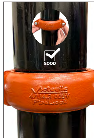
PHOTO 4 (ACCEPTABLE) – HOUSINGS' KEYS ALIGNED WITH PIPE GROOVES
